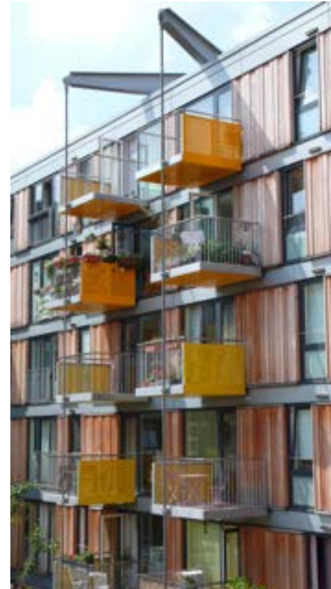
Figure 4.13: Example of a tall building with high quality materials and detailing
